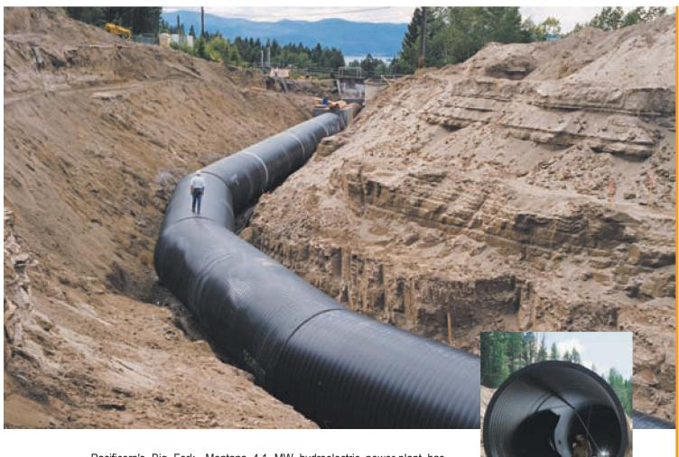
Pacificorp's Big Fork, Montana 4.1 MW hydroelectric power plant has been in service for over 100 years. Weholite was selected to replace a woodstave penstock feed line that parallels the Swan River. After many years of service, in 2000, a failure of the woodstave pipeline caused a washout into the scenic Swan River, along a section of the river that is popular for canoeing and whitewater rafting. The plant's electrical output was cut in half, pending replacement of the pipeline.
